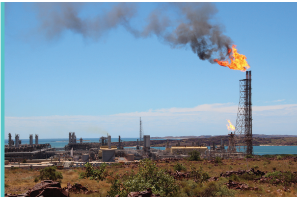
Woodside's North West Shelf Karratha Gas Plant
